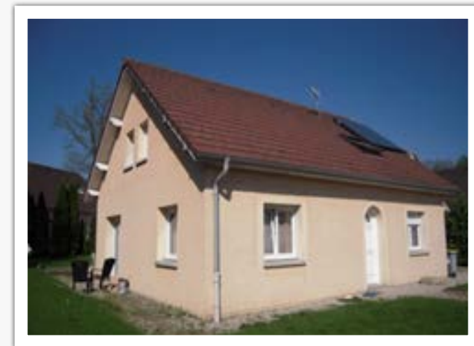
Baume-les-Dames, Doubs, Source Efflogis
